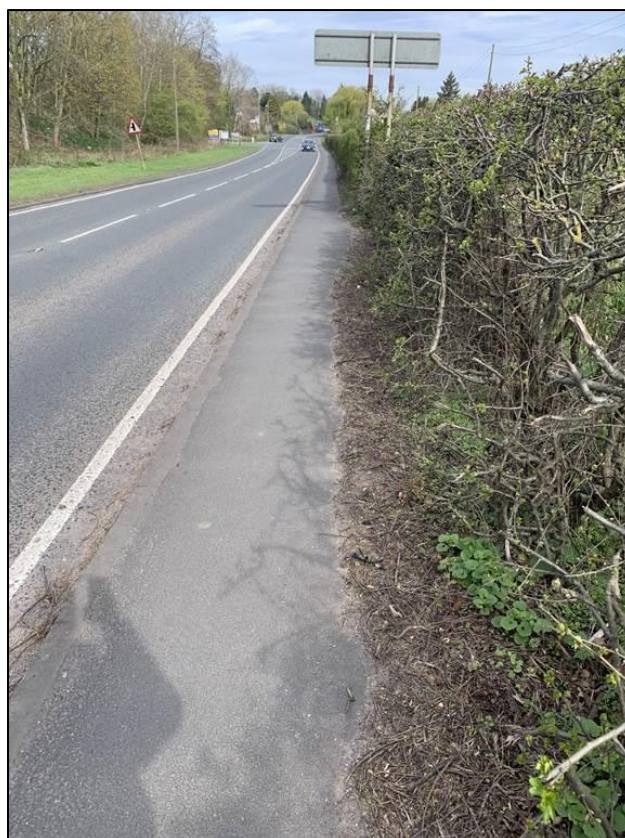
Footway narrowed by overgrown vegetation
