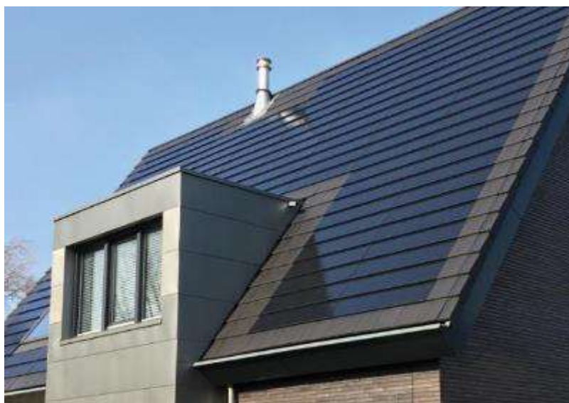
Solar tiles are flush with the roof and less obtrusive than solar panels (image credit Crest BST)
