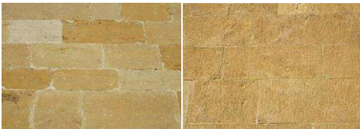
Stone for new buildings must match the colour and style of existing buildings. Here, two examples show ashlar walls in Broadway, laid to produce tight, thin joints. Often the face of the stone will be rubbed plain, though the wall on the right shows stonemason's marks faintly visible. Ashlar walls are particularly appropriate for larger, more formal houses.
