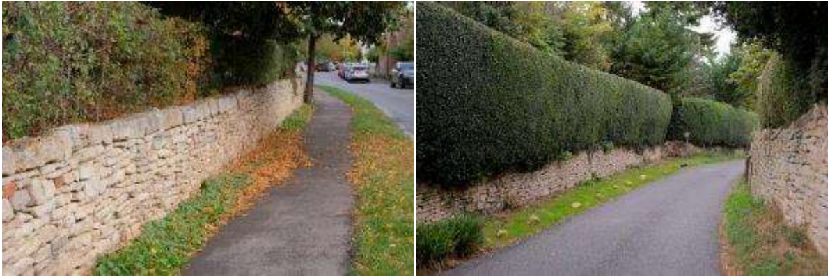
A footpath-facing boundary wall in Bredon combines a dry stone wall and hedge (left) and a dry stone wall and hedge with a generous green verge (right) creates a pleasant rural lane in Bredon's Norton
