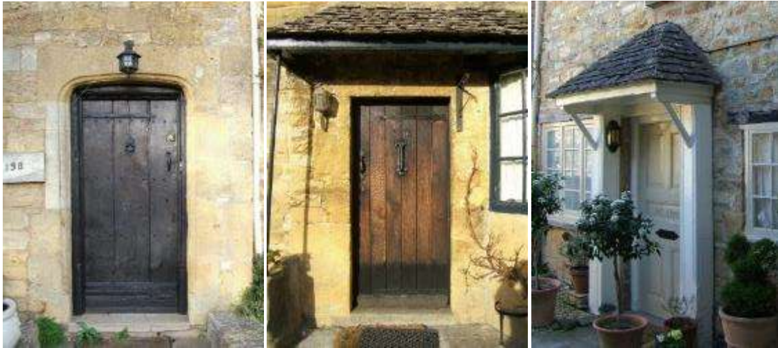
Timber panelled doors in a vernacular style in Broadway
