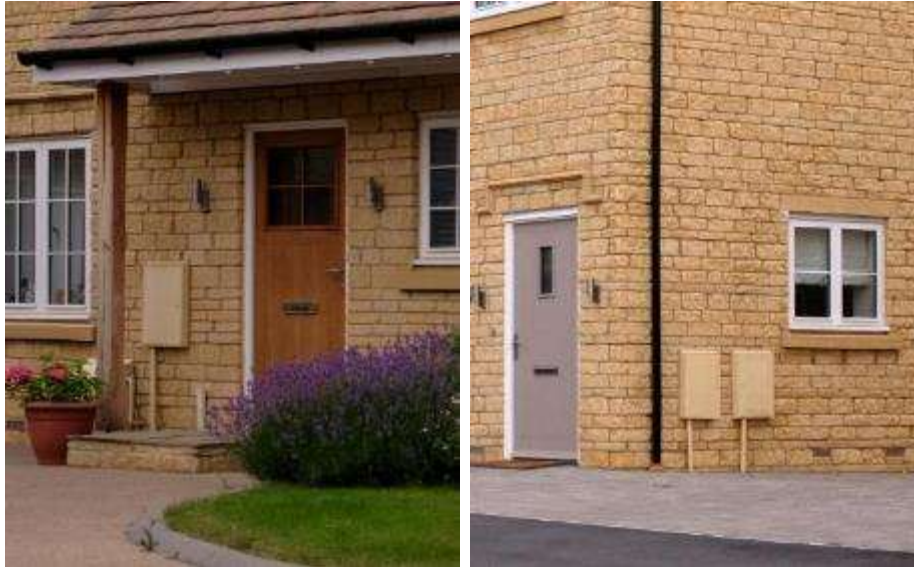
Examples of inappropriate, overly conspicuous meter box placement. The example on the left should be lower and further from the door, while the example on the right should be lower and further back along the driveway. The requirement for border planting in this design code would aid both these situations.
