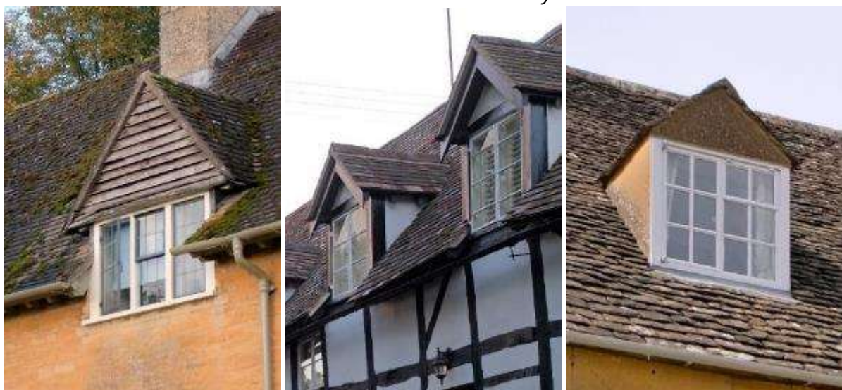
A large wall dormer in Overbury (left), dormers in Elmley Castle (centre) and a simple dormer in Broadway (right)
