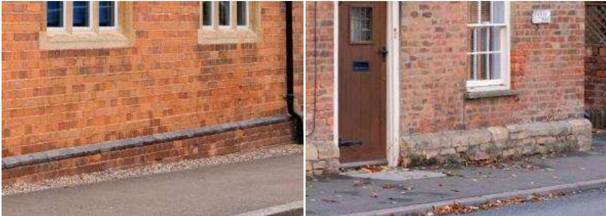
A brick plinth in Ashton under Hill (left) and a substantial stone plinth on a brick building in Kemerton (right)
