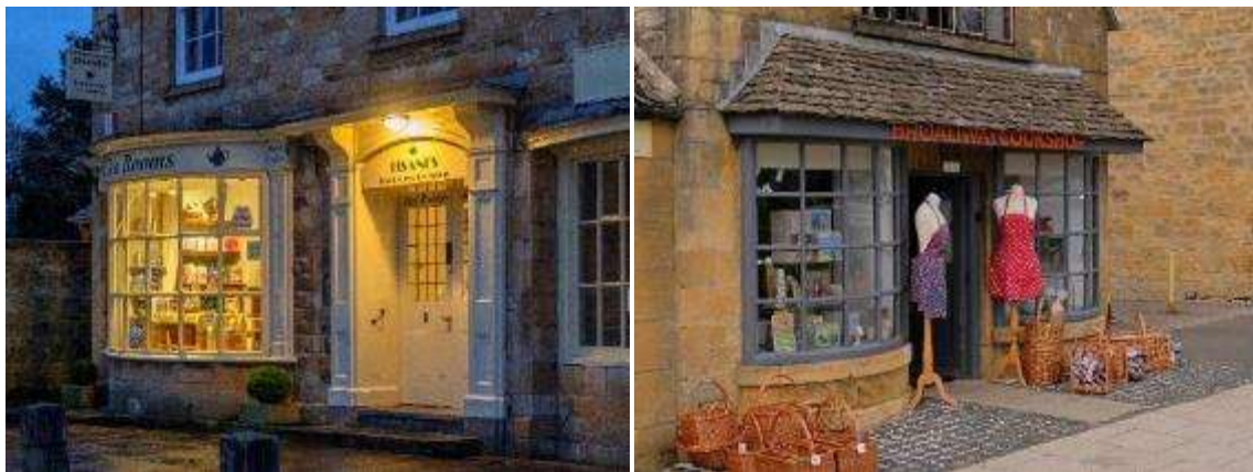
Shopfronts in Broadway with lettering integrated into the curved window (left) and into the fascia (right)
