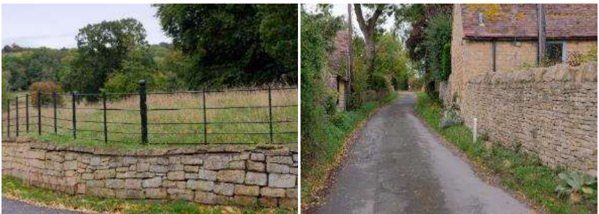
A combination stone wall and estate fence in Bredon's Norton (left) and a stone wall along a narrow rural lane in Westmancote (right)
