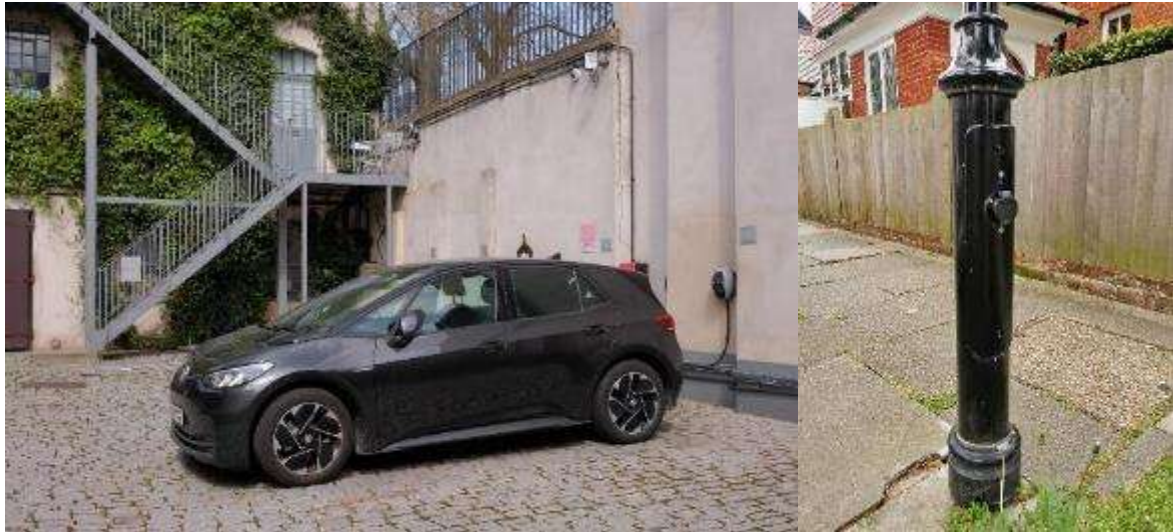
A discreet building or wall-mounted EV charger is an appropriate option for courtyard parking (left), or a charger can be included in a lamp post or bollard (right)
