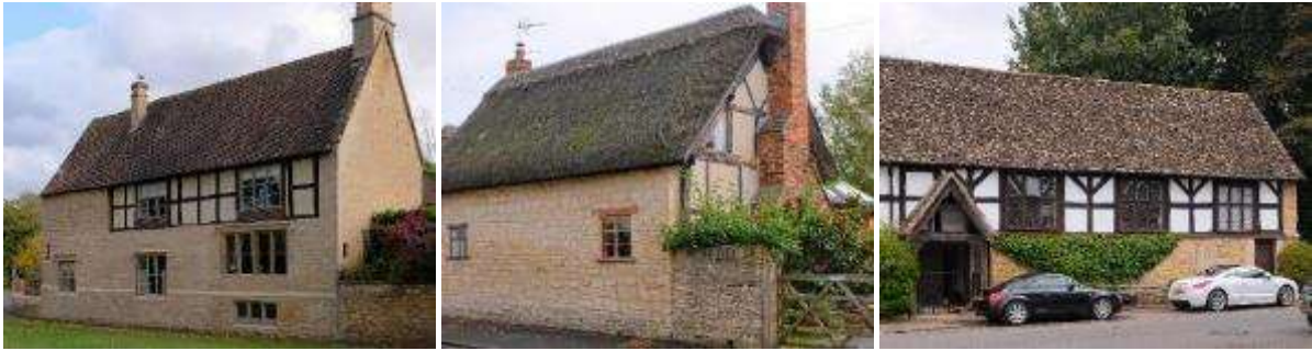
Hybrid timber frame homes with stone and brick walls in Beckford (left), Bredon (centre) and Elmley Castle (right)
