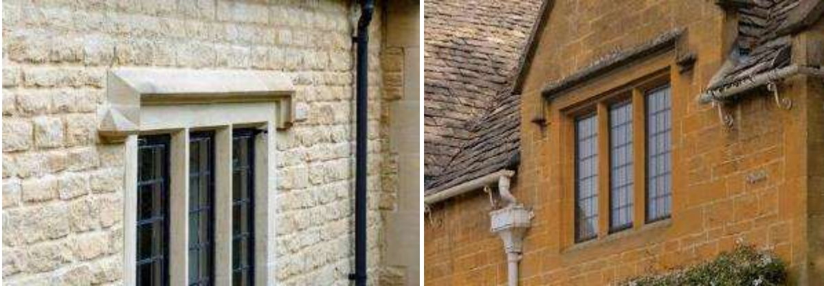
A new stone hood mould over a window (left) and an example in Broadway (right)
