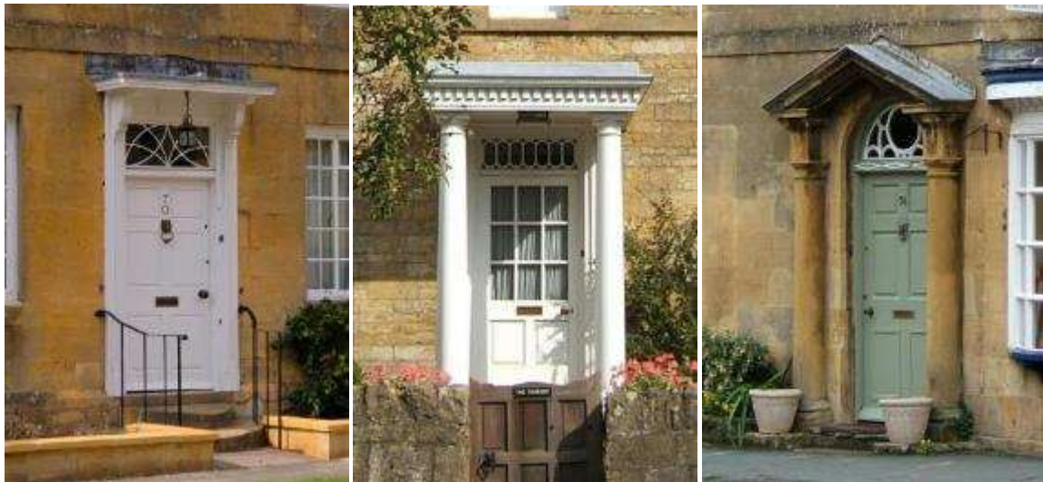
A classical door and door canopy or porch can be an appropriate choice for a formal, classically design house, such as these Broadway examples
