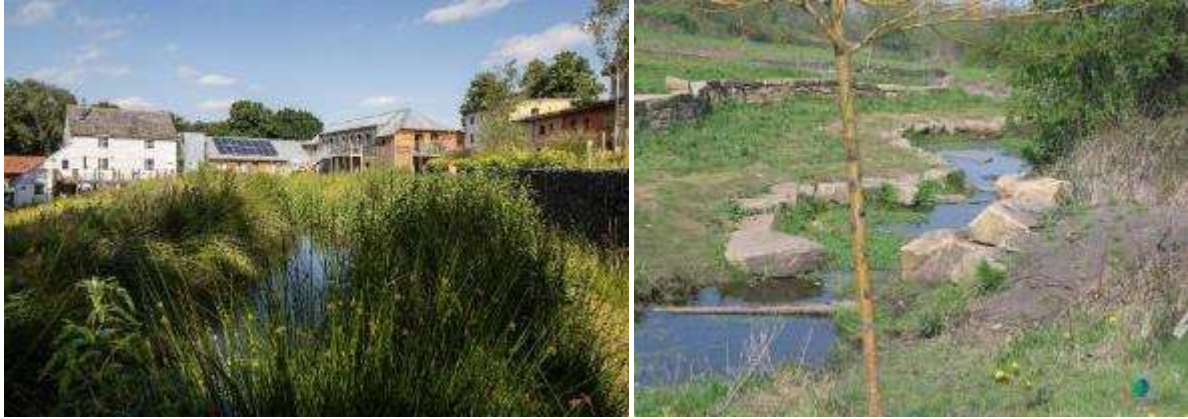
SuDS at Cannock Mill Cohousing (left) and a stone-lined narrow basin at The Manor, Sheffield (right, image credit Susdrain) are examples of SuDS appropriate for a rural development
