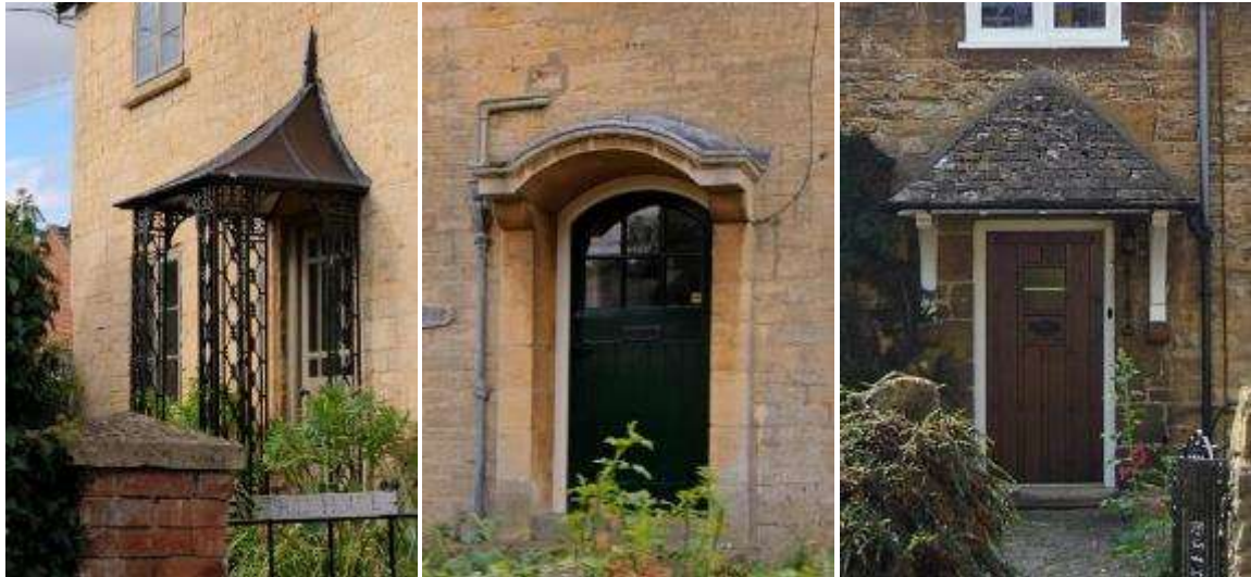
A cast iron porch in Kemerton (left), an Arts & Crafts door and canopy in Conderton (centre) and a large canopy in Broadway with timber brackets well suited to a cottage aesthetic (right)
