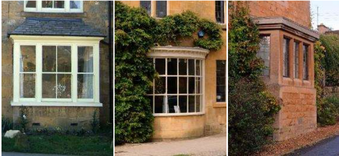
Victorian bay window in Broadway (left), a delicate Georgian bay window in Broadway (centre) and a stone mullioned example in Overbury (right)
