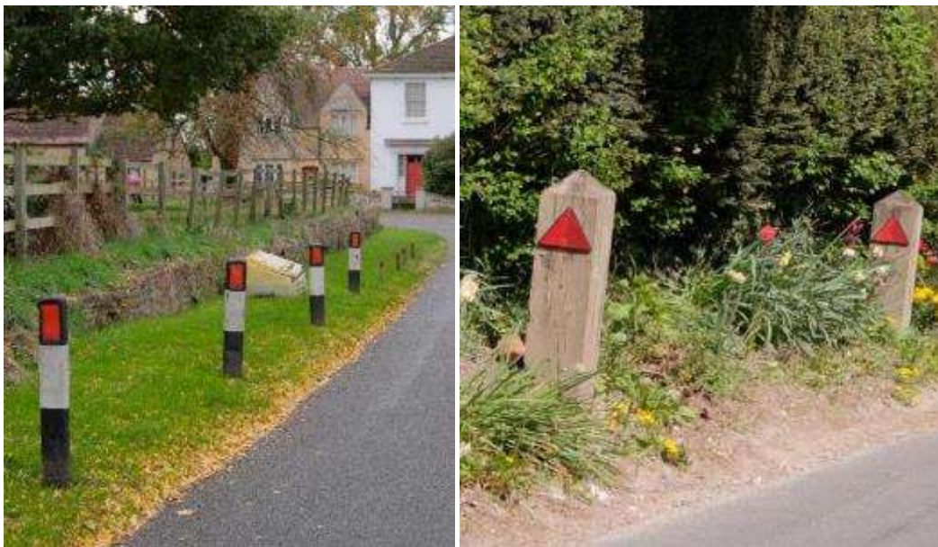
Plastic bollards must not be used (left). Instead, in villages and rural areas, timber bollards are a more sympathetic option (right).
