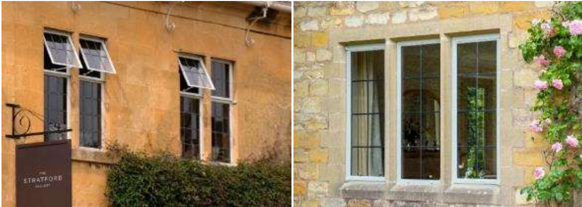
A portion of the window can be a top hung casement window, as this example in Broadway shows (left). New casement windows (right, image credit The Cotswold Casement Company)
