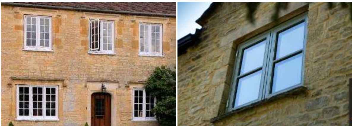
Casement windows on a house in Ashton under Hill (left) and timber/aluminium composite casement windows (right, image credit Enlightened Windows)
