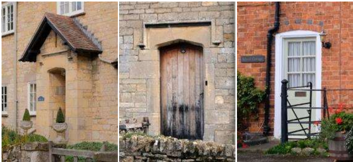
A substantial stone porch in Kemerton (left), a panelled door in Overbury (centre) and a glazed door in Beckford (right)
