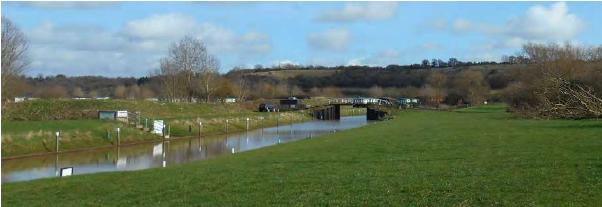
Photo 5 - Bridge over navigation at George Billington lock (public footpath)
