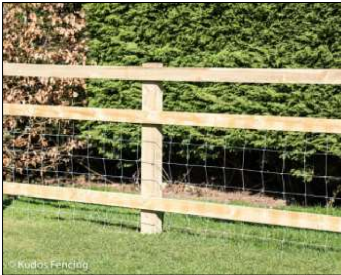
Plate 6: Example of post and rail fence with wire mesh (Source: Kudos Fencing )
