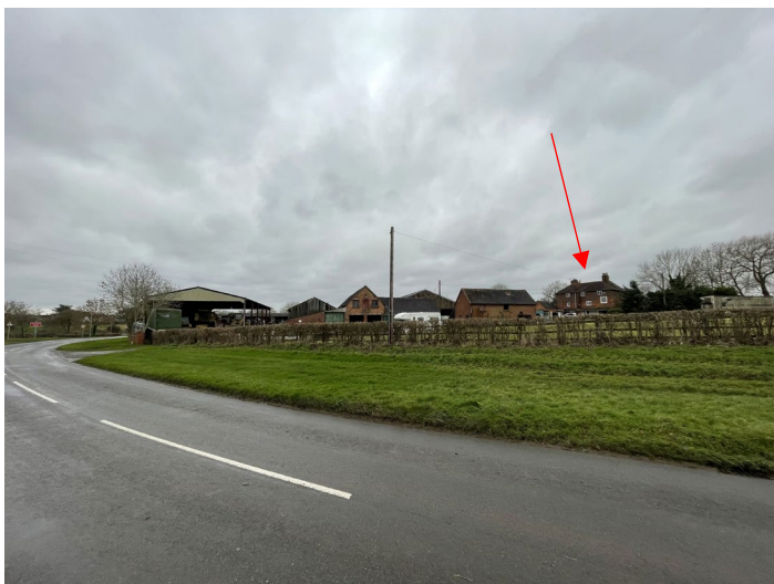
Plate 13 Looking south-west to the Tapenhall Farm complex from Dilmore Lane
