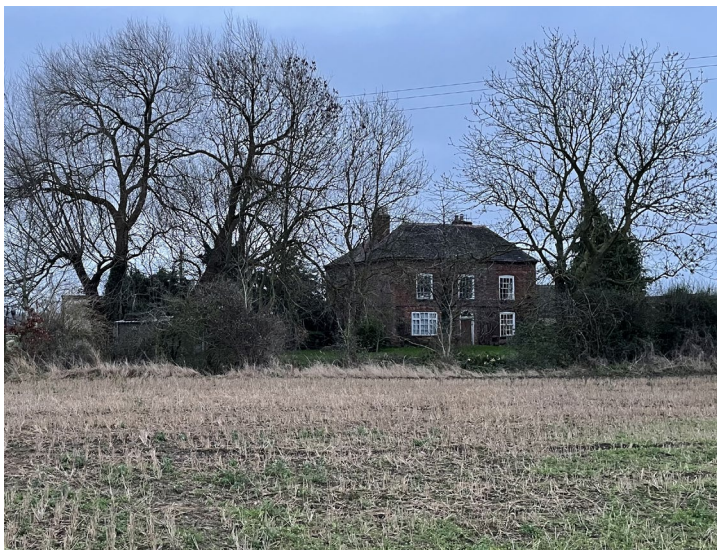
Plate 6 Looking south-east to the primary western façade of Tapenhill Farmhouse
