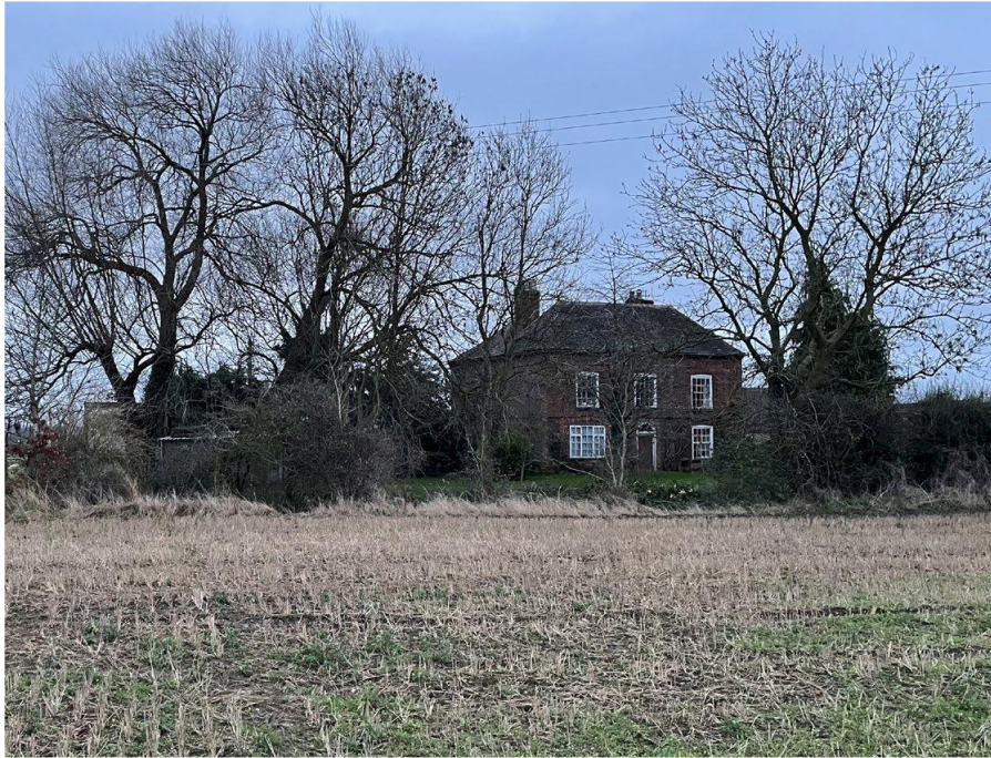
Plate 1 Looking south-east to the primary western façade of Tapenhill Farmhouse
