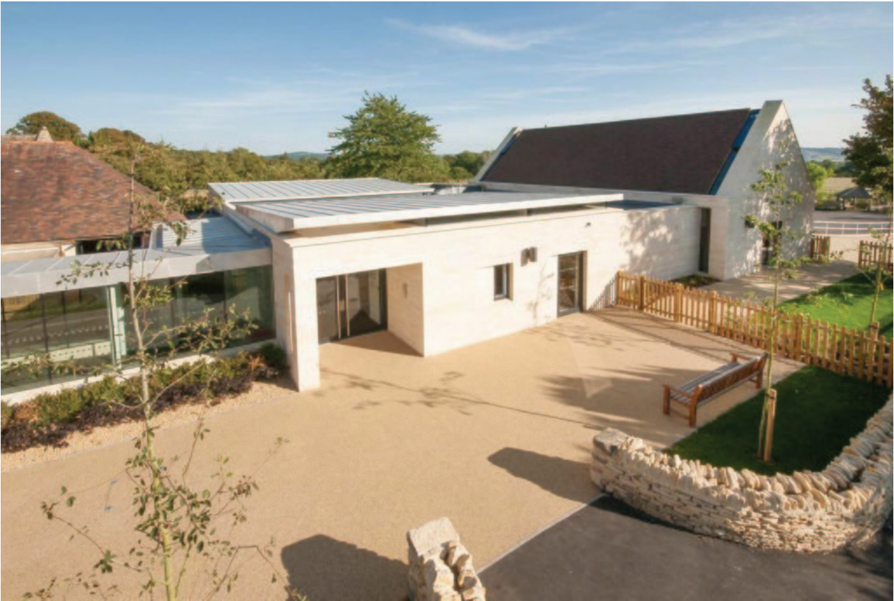
Overbury First School
